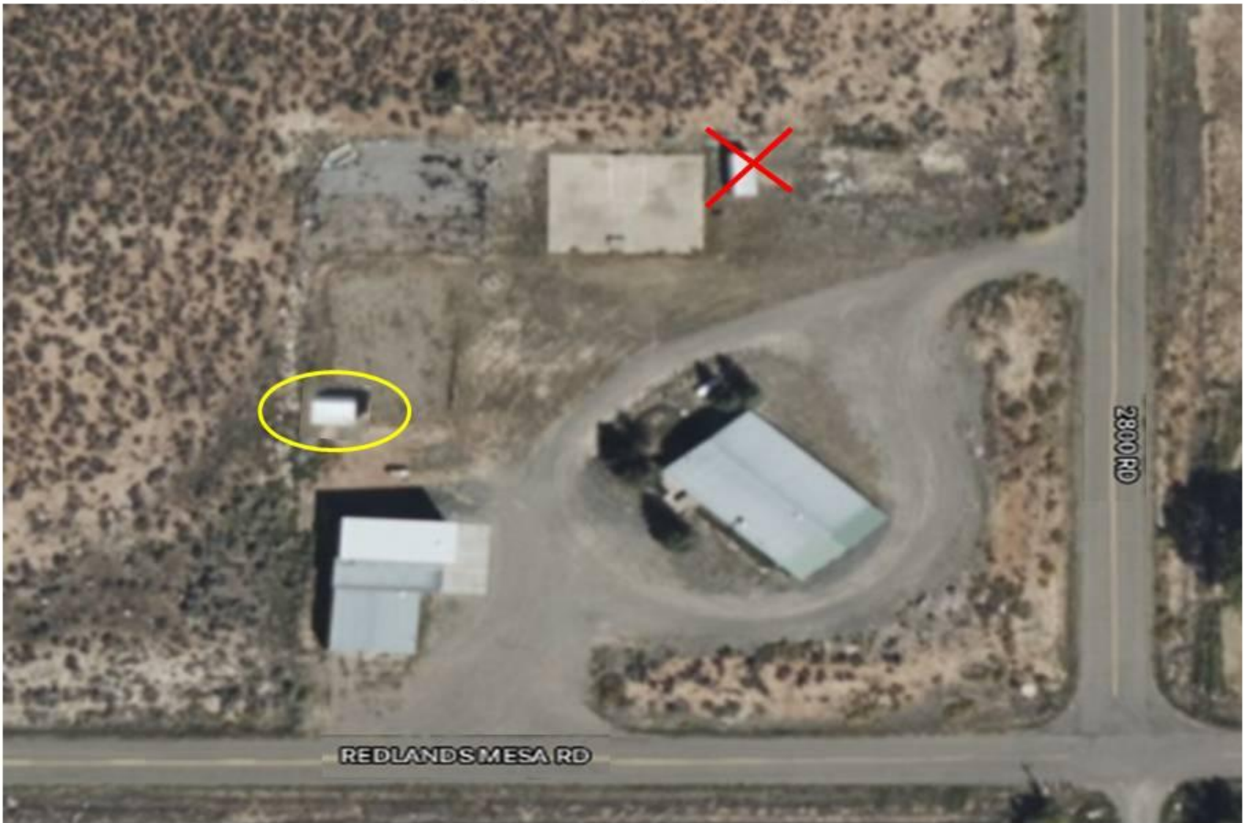
Current GIS Image RMG #487 and Redlands Mesa VFD – Showing proposed & Doug Fritz endorsed, storage building relocation
